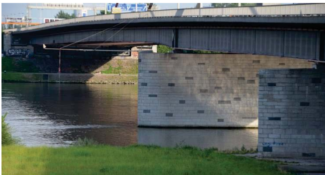
Figure 3: Voest-bridge with existing bridge piers
