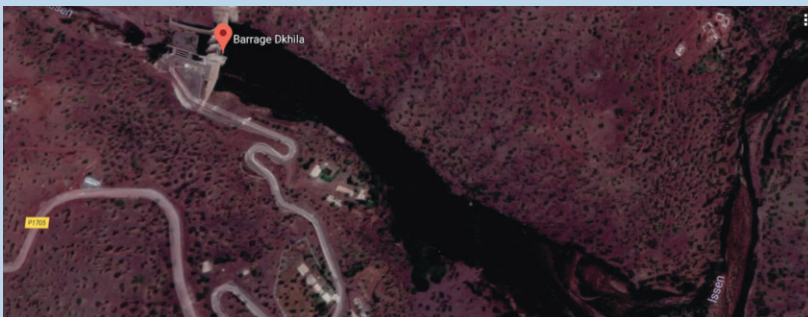
Figure 3. Dkhila dam (service year: 1986, height: 37 m, initial reservoir capacity: 0.7 Mm 3 , sedimentation rate: 0.03 Mm 3 /per year), Issen River, Souss Massa Draa basin (Google Earth)
