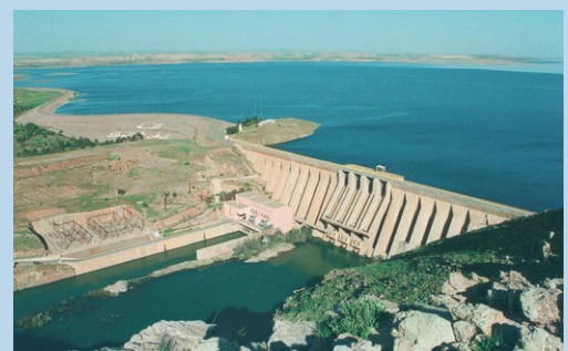
Figure 4. Al Massira dam (service year: 1979, height: 82 m, initial reservoir capacity: 2,785 Mm 3 , sedimentation rate: 2.3 Mm 3 /year), Oum Rbia River, Oum Rbia basin
