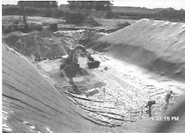
Figure 4: Filling the basin with sand and build-up of the clay levee
