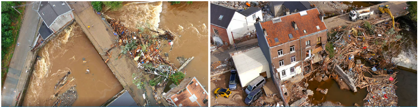
Figure 3 | Role of debris in damming part of the river section, affecting flow depths upstream and leading to flow contraction, scour, and high local damages (river Vesdre, upstream of Verviers). Credit: J. Mawet
