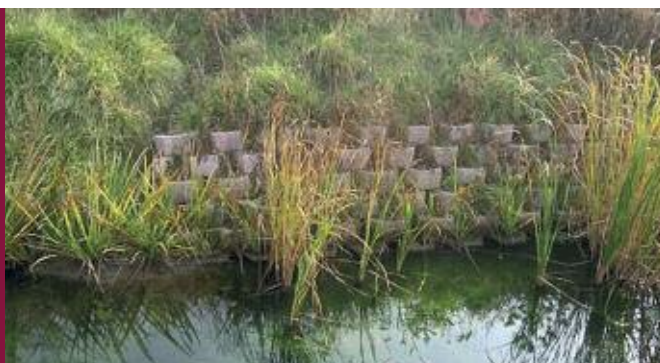
Figure 3. Vegetated block slope protection
