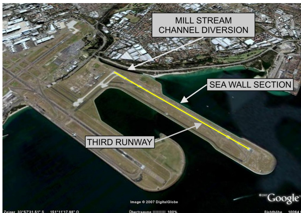
Figure 1. The runways of Sydney's Kingsford Smith International Airport with Millstream Diversion and Seawall.
