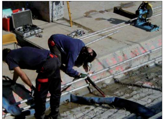
Figure 4: Placing of the air pipes
