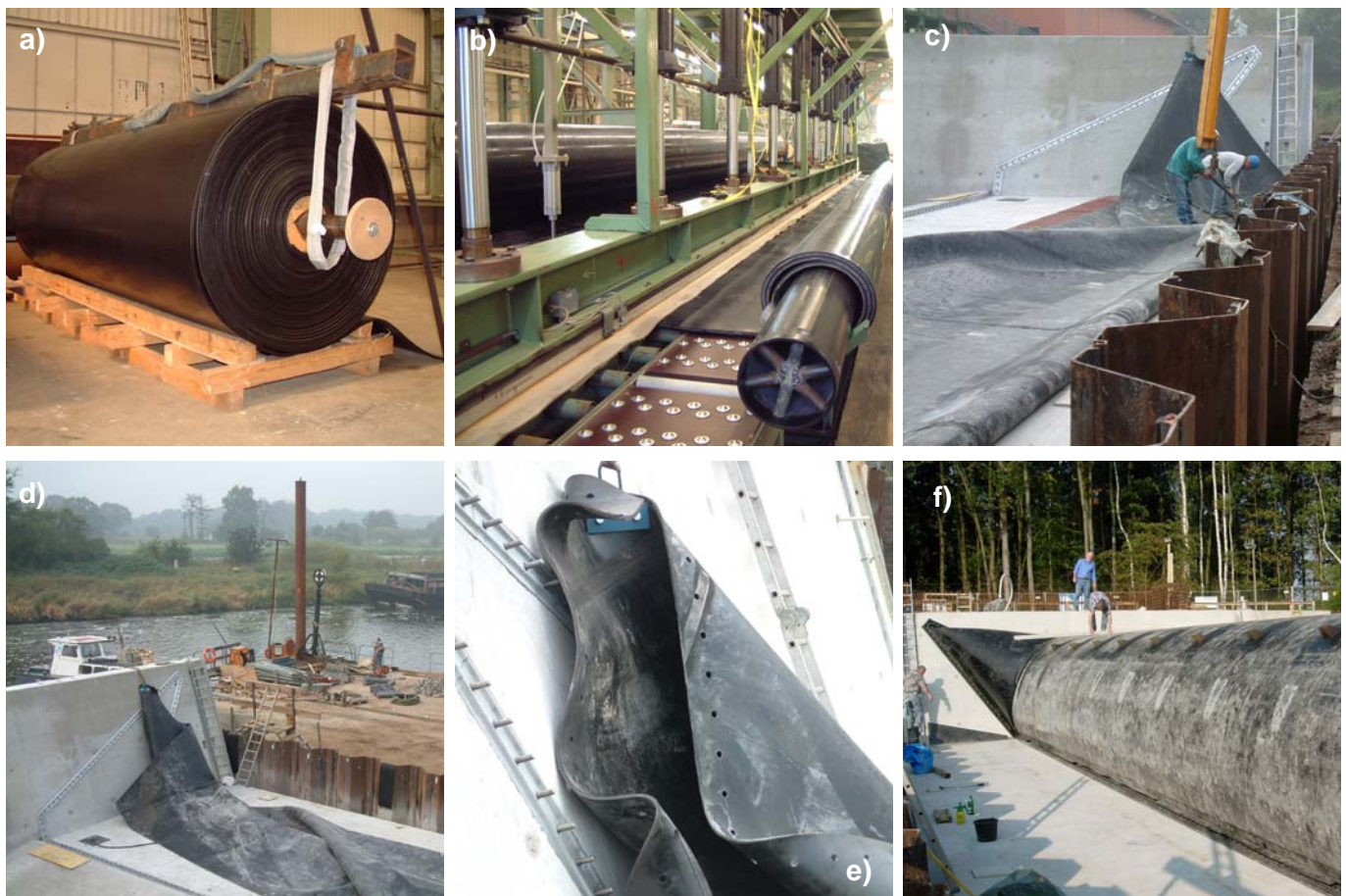
Figure 1: Weir Marklendorf on the River Aller: a) Membrane after calendaring b) Joining the sheets c) to e) Installing the rubber membrane in October 2005 e) Pressure test
