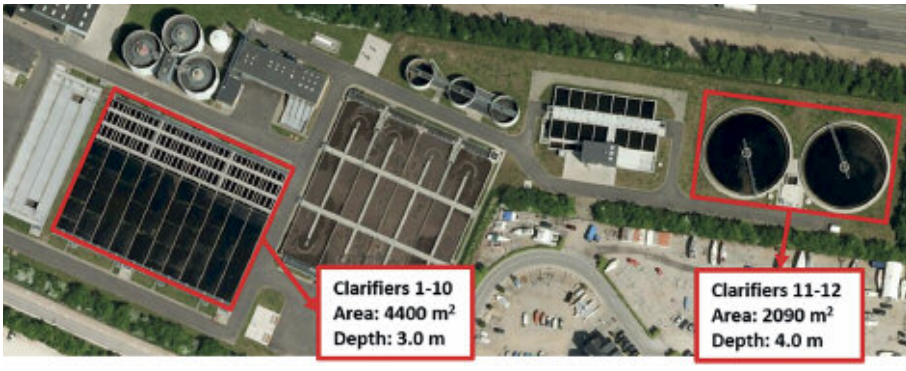
Figure 6. Marselisborg WWTP, Aarhus, Denmark is equipped with two clarifier lines
