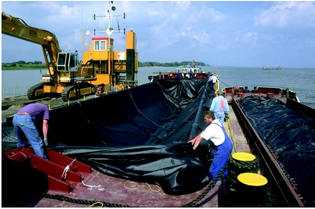
Figure 8: Large geosynthetic containers (Photo: Colcrete - von Essen)
