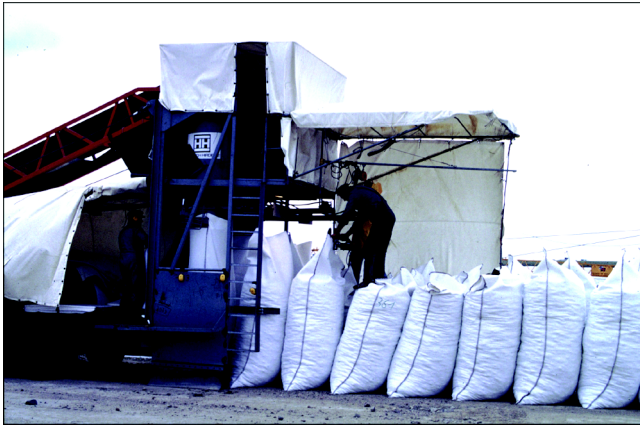
Figure 7: Filling plant for geosynthetic containers
