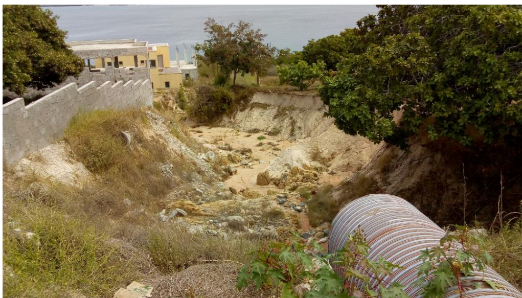
Fig. 8. Erosion due to storm water runoff in Nacala City.
