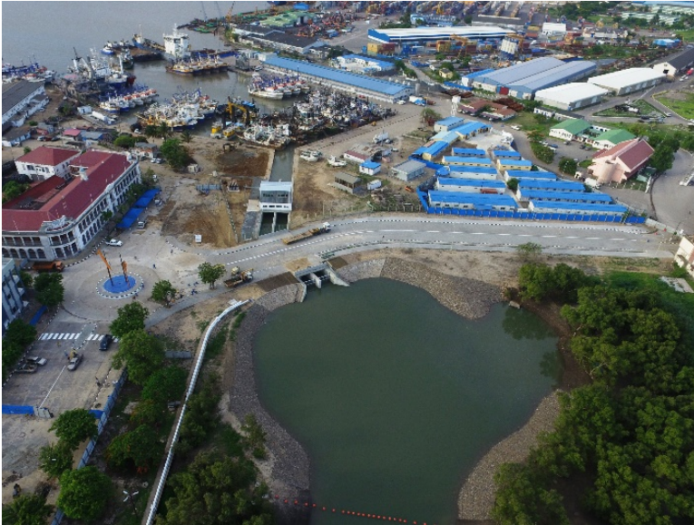
Fig. 2. Aerial photograph of the Chiveve river mouth including the new flood barrier.
