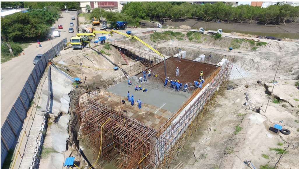
Fig. 3. Construction of the drainage channel upstream of the tidal outlet.
