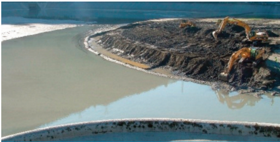
Figure 4. Cleaning operation at the Longefan reservoir, France. (Courtesy: EDF)
