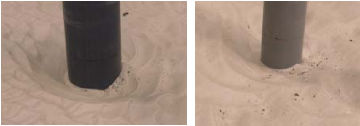
Figure 2 Photo taken after execution
