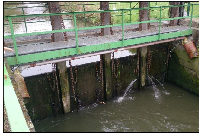
Figure 5. Detailed view on the wooden boards of the small weir at Geraardsbergen. Chains are attached to hoist the boards. (picture taken 29/04/2016)
