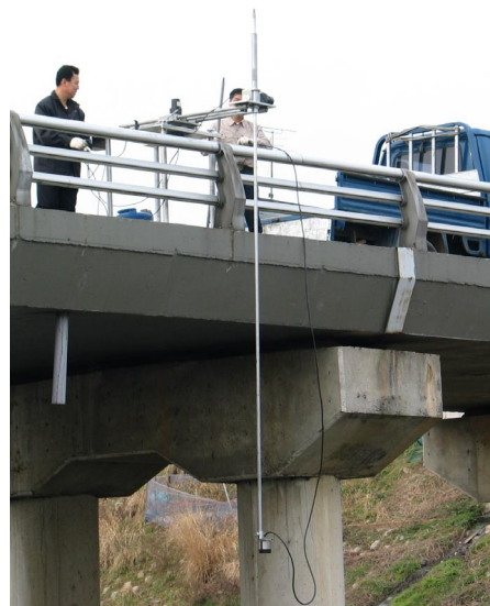
Figure 5. Scene of preparation for measuring pier scour
