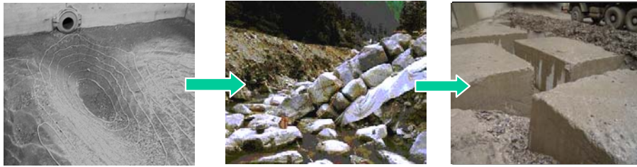
Figure 1: Scour in alluvial bed downstream of a diversion tunnel outlet (left), riprap protection on a river bank (middle), concrete prisms as erosion protection (right)
