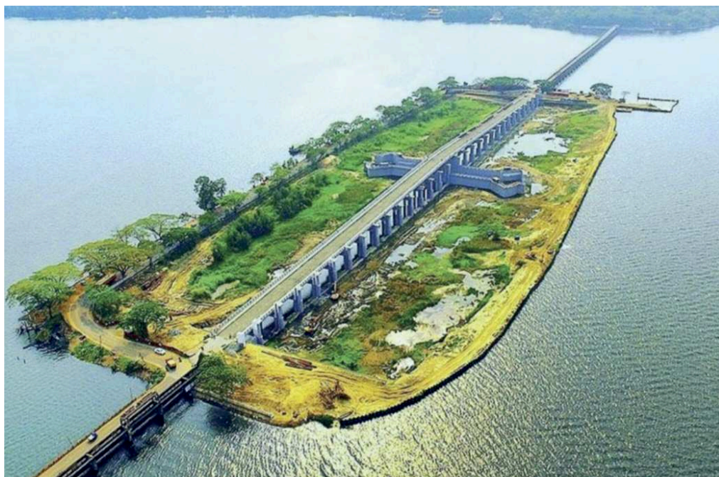
Figure 1. View of the Thaneermukkom bund
