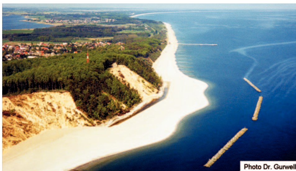
Fig. 8: System of detached breakwaters at Streckelsberg/Usedom
