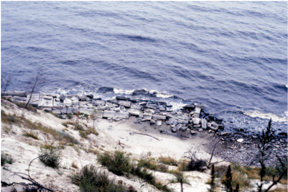
Fig. 7: Destroyed Streckelsberg Wall
