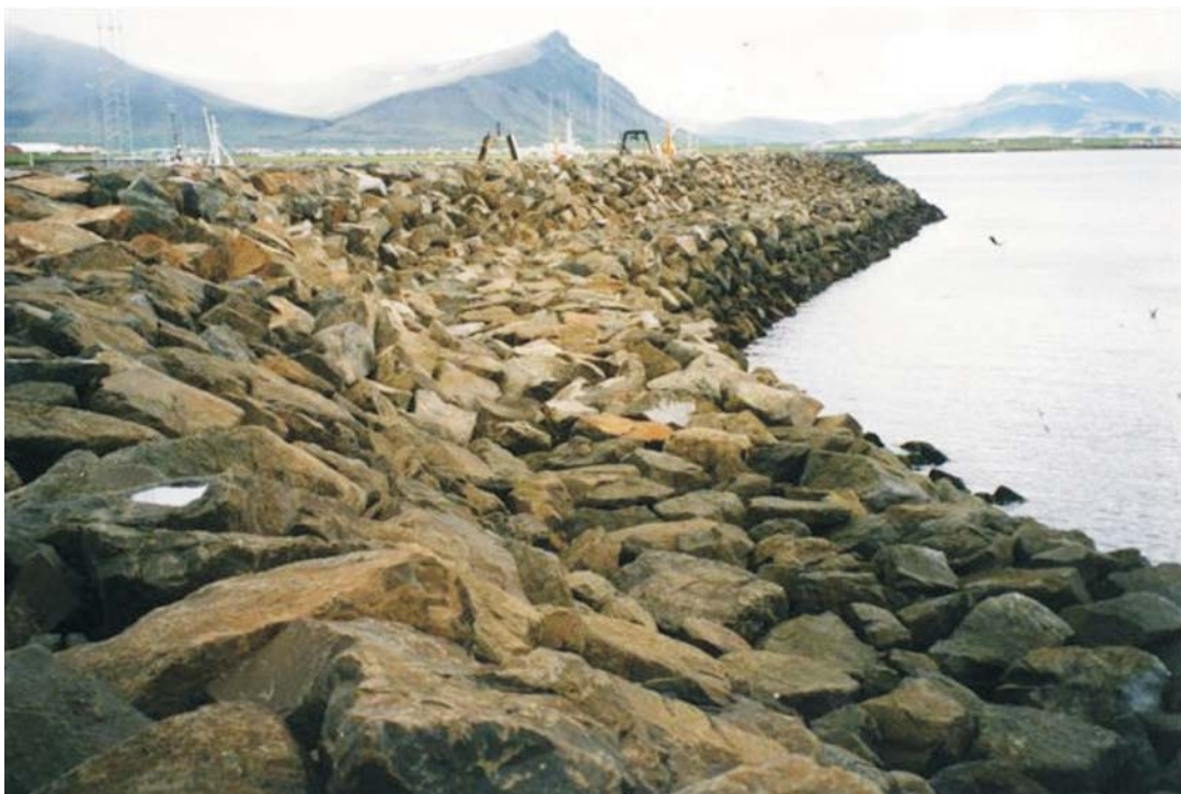
Fig. 6.7: Icelandic Berm breakwater
