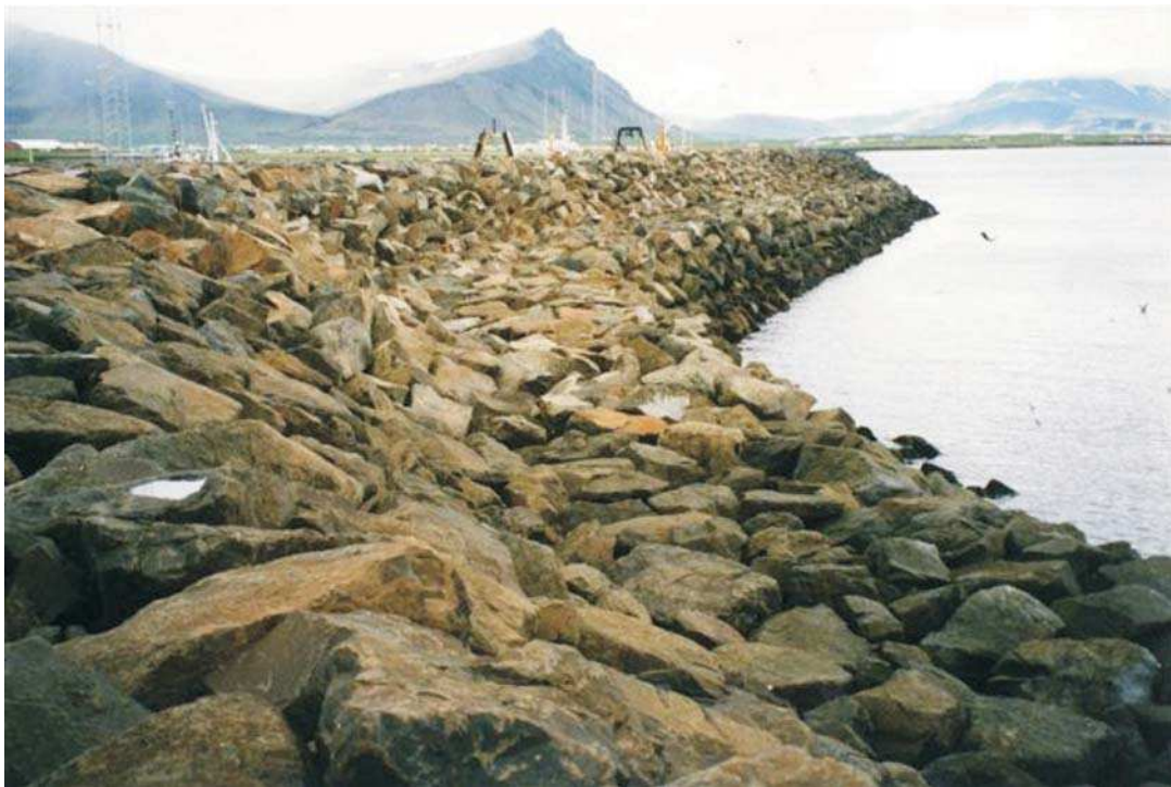
Fig. 6.7: Icelandic Berm breakwater
