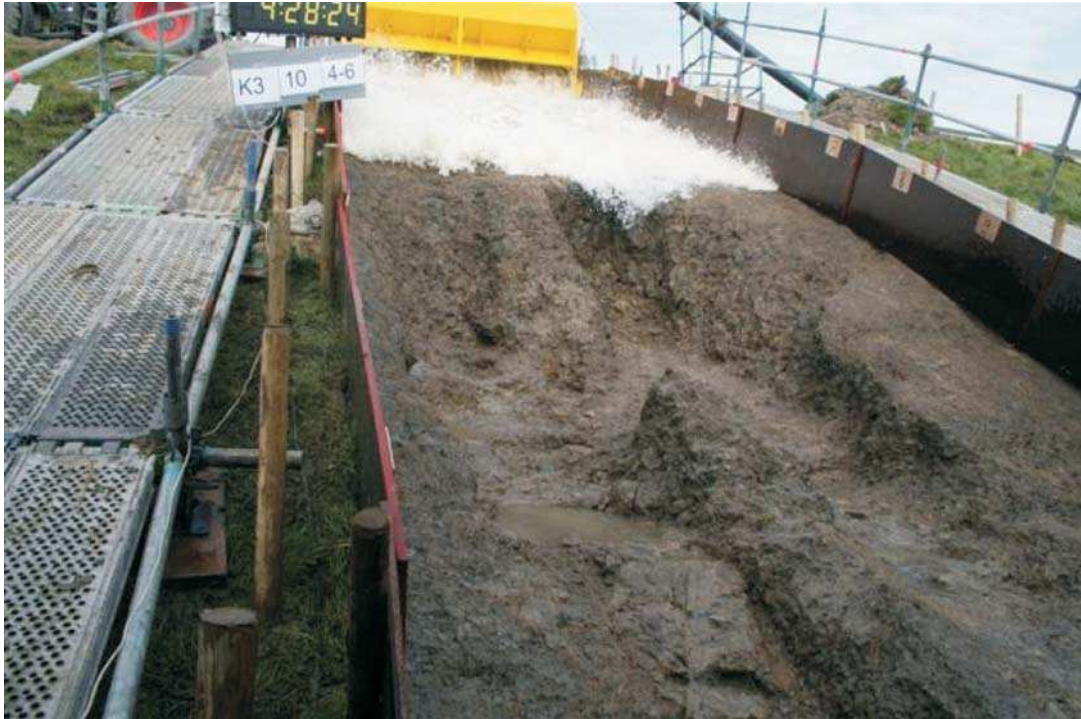
Fig. 3.2: Wave overtopping test on bare clay; result after 6 hours with 10 l/s per m width
