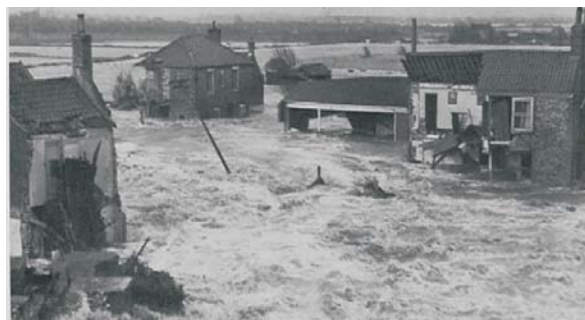
Fig. 2: Flooding in Lincshire during the 1953 storm surge
