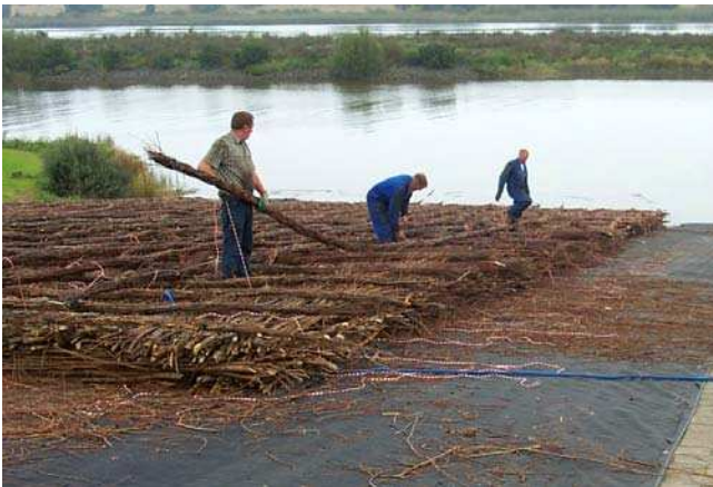
Fig. 8 Preparing a fascine mattress (including additional brushwood layer)
