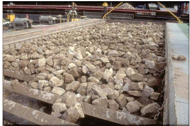
Fig. 10 Stone dumping pontoon
