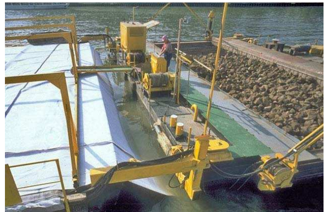
Fig. 11 Geotextile filter placement under water
