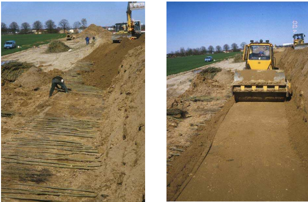
Figure 5: Placing plants on a berm, covering them with soil and compacting it
