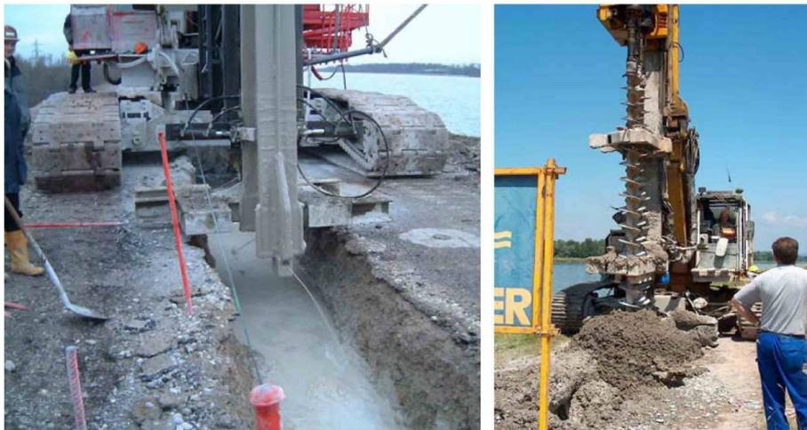
Figure 6: Installation of a cut-off wall (left : diaphragm wall, right : mixed-in-place wall)
