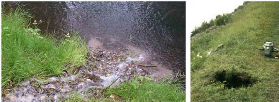
Figure 4: Damages due to internal erosion
