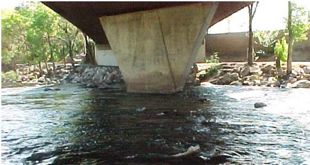
Figure 2. Kuenzli Street Bridge Pier
