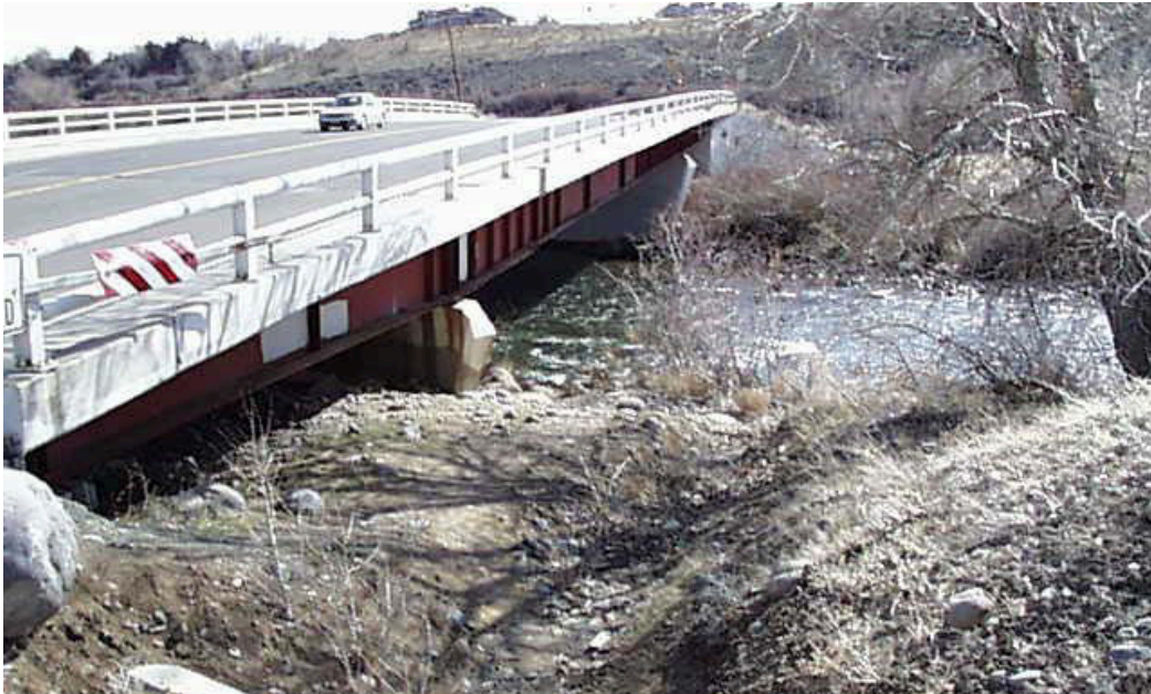
Figure 4. Mayberry Drive Bridge
