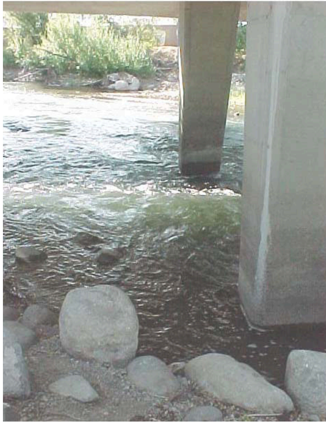
Figure 1. Kietzke Lane Bridge Piers
