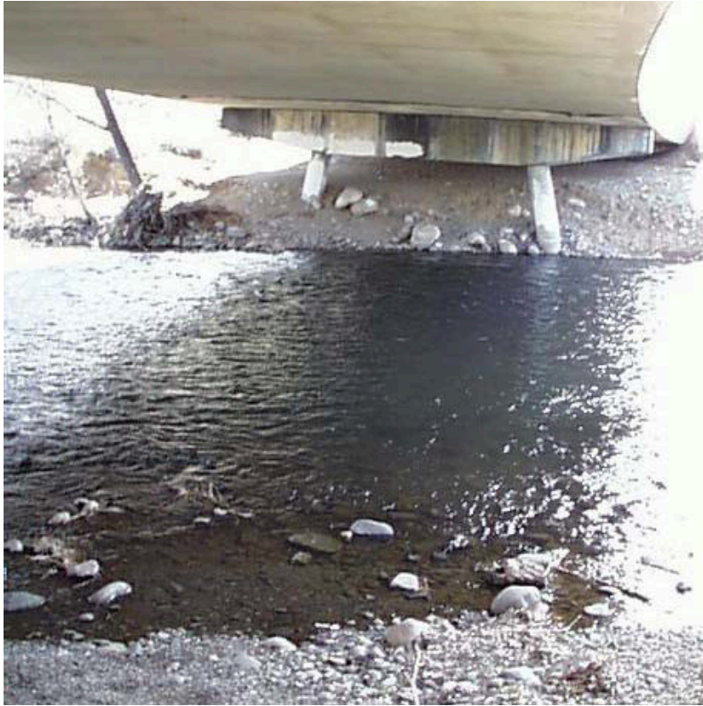
Figure 3. Keystone Avenue Bridge
