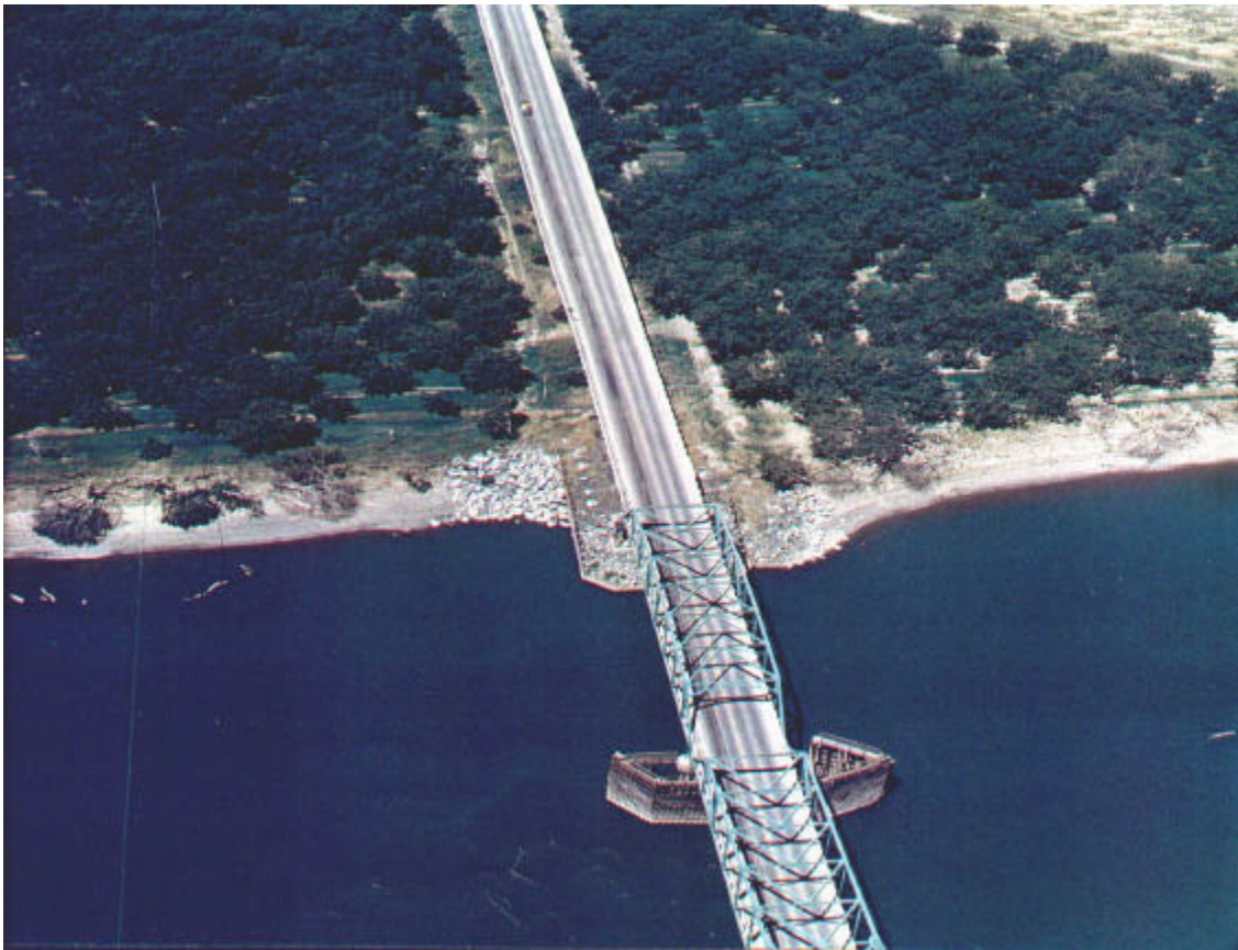
Figure 5: Repair work at pier 107 done in 1997
