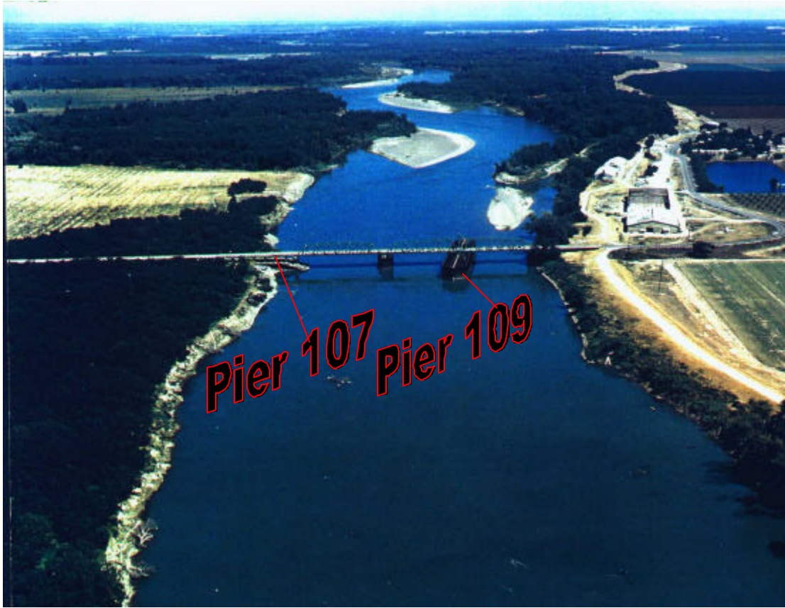
Figure 1: A bird's eye view of the bridge location
