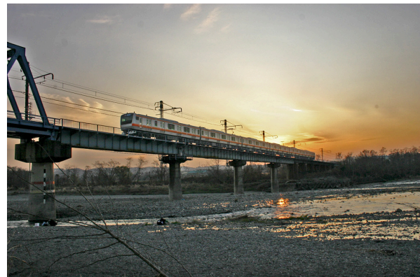
Fig.1 The view of bridge A
